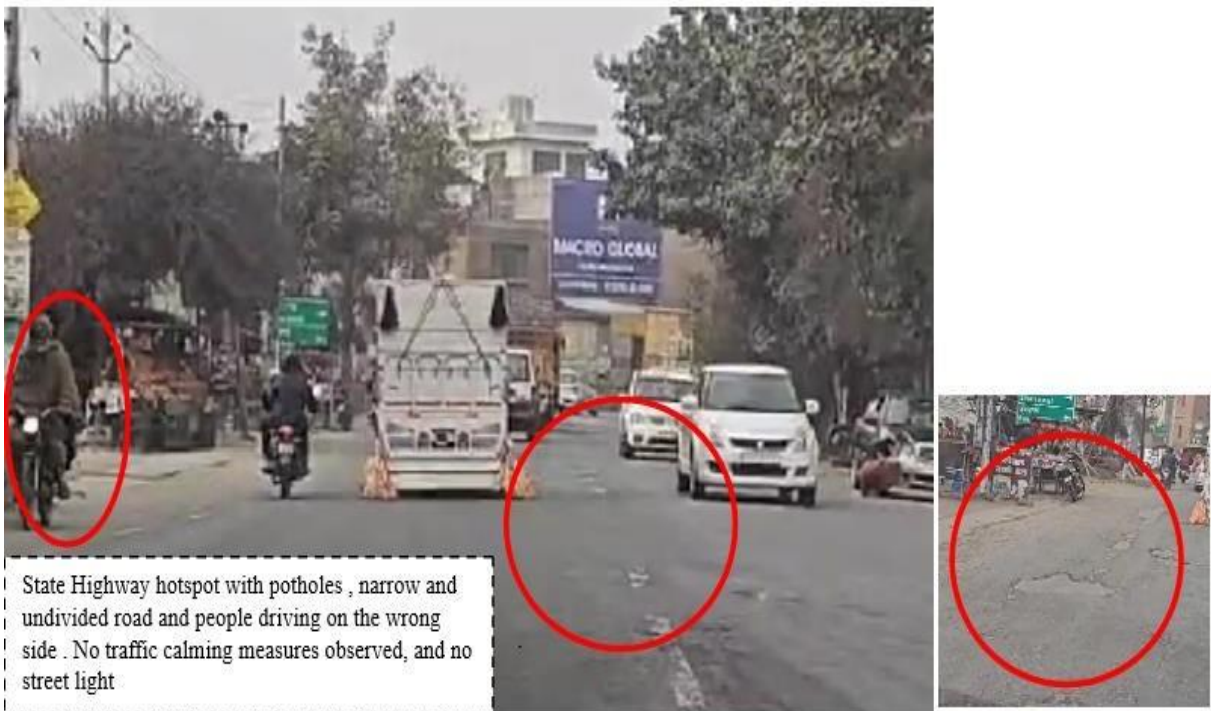
Figure 3.17 Observed potholes and road condition highlighted in red
